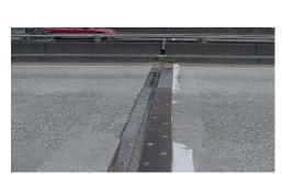
414 – Bolt Down Sliding Plate with Springs
