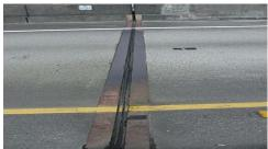
406 - Compression Seal/Steel Header
