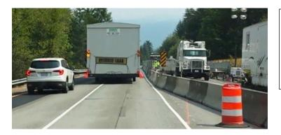
Oversized truck freight example; modular home straddling both lanes on Interstate 90 at a bridge rehabilitation work zone with a reduced traveled way. *Source*: WSDOT
