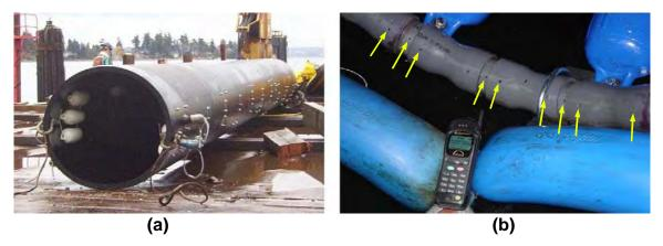
Figure 2: (a) Photograph of bubble curtain sheath during construction. (b) Photograph of one of the 3"diameter aerating tubes affixed to the inside of the bubble curtain — yellow arrows indicate the positions of the 1/8" diameter air holes.
