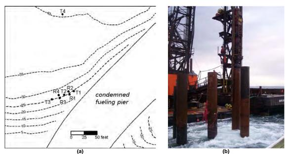
Figure 1: (a) Plan view diagram showing the pile locations at the test site with depth contours in feet. (b) Photograph of the steel piles (R1-R4 and T2) and the pile driving hammer. The hammer was suspended over pile R2 and the crane barge can be seen in the background. The froth on the water was caused by the active bubble curtain.
