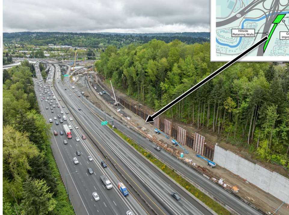
Looking northeast at soldier pile and tieback wall construction along northbound I-405.
