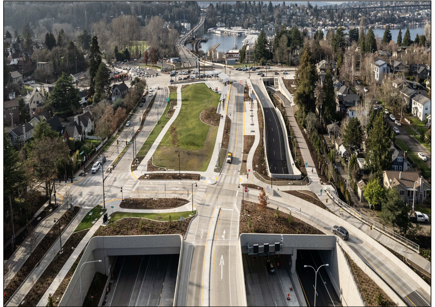
View of the completed Montlake Lid from above.
