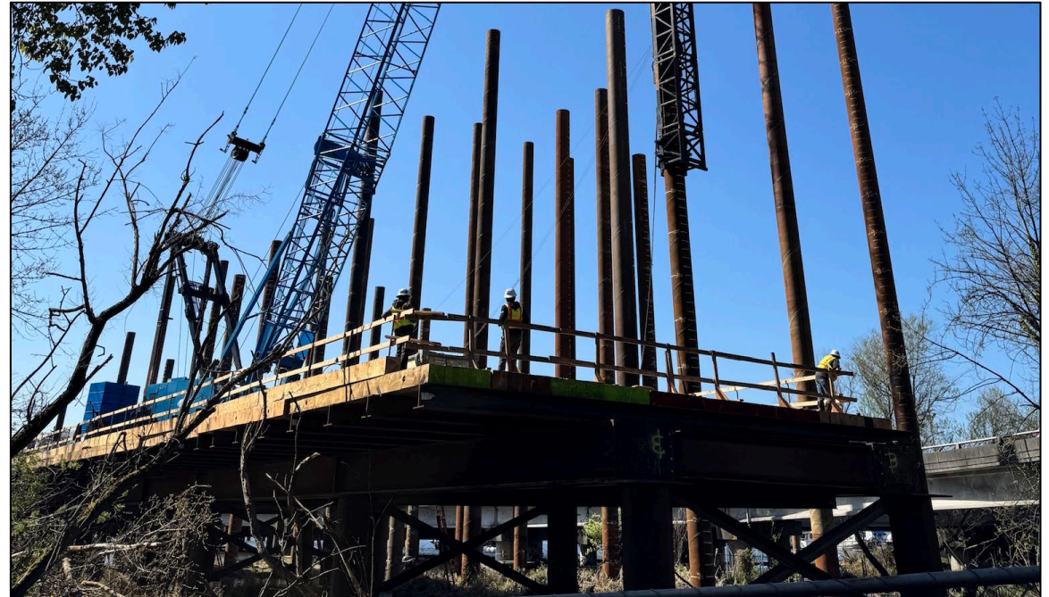
Crews installing piling in Portage Bay during the day.
