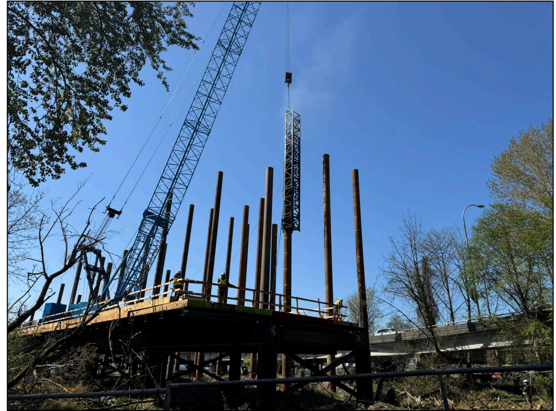
Crews installing piles near Portage Bay.
