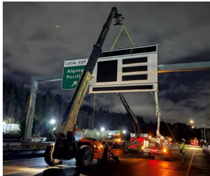
New toll sign installation for destination pricing
