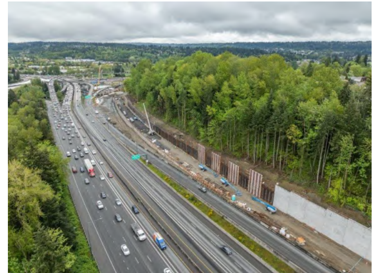
Pouring fascia on the retaining wall along the east side of I-405
