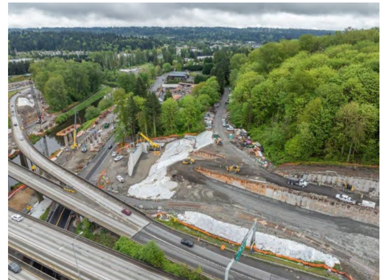
Prep to set girders across the Sammamish River for new northbound I-405 on-ramp to eastbound SR 522
