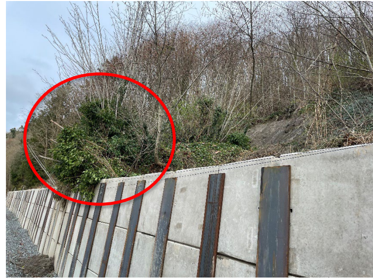
Landslide behind catchment wall – Mukilteo, WA
