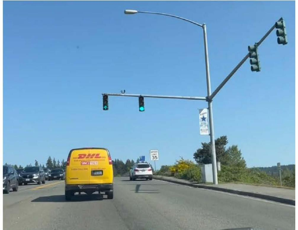
Olympic Region Figure 2 - Northbound State Route 3 at Kitsap Mall - Upgrading Signal to Through Arrow Before and After
