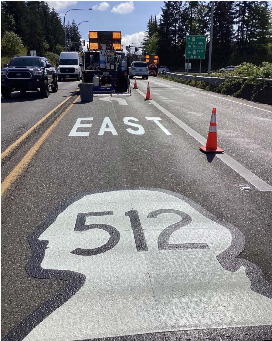
*Olympic Region Figure 1 – State Route 512 Example of Improved Pavement Marking with Direction and Route Shield*
