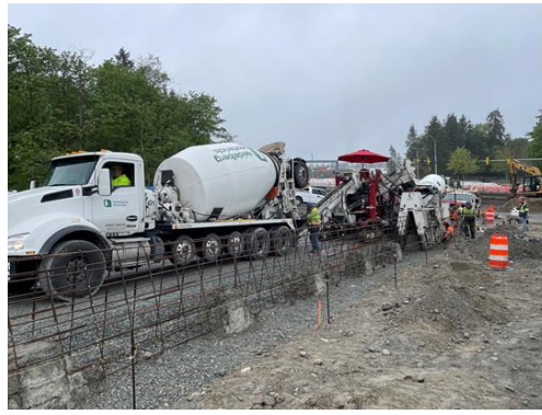
Crews placing concrete barrier for the new eastbound SR 516 to northbound I-5 ramp.
