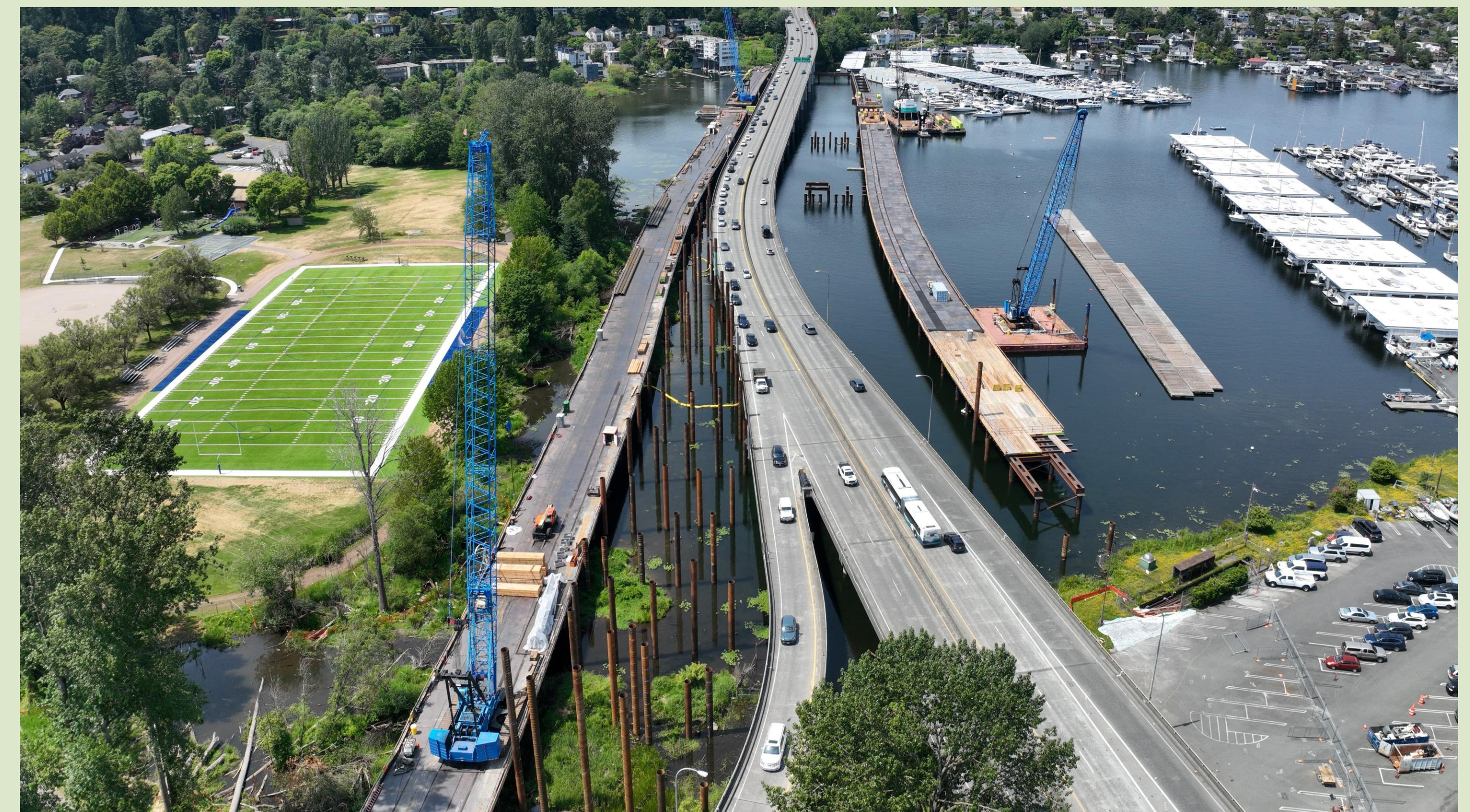
The steel piles between the existing bridge and the work trestle will support a new temporary eastbound off-ramp to Montlake Blvd.
