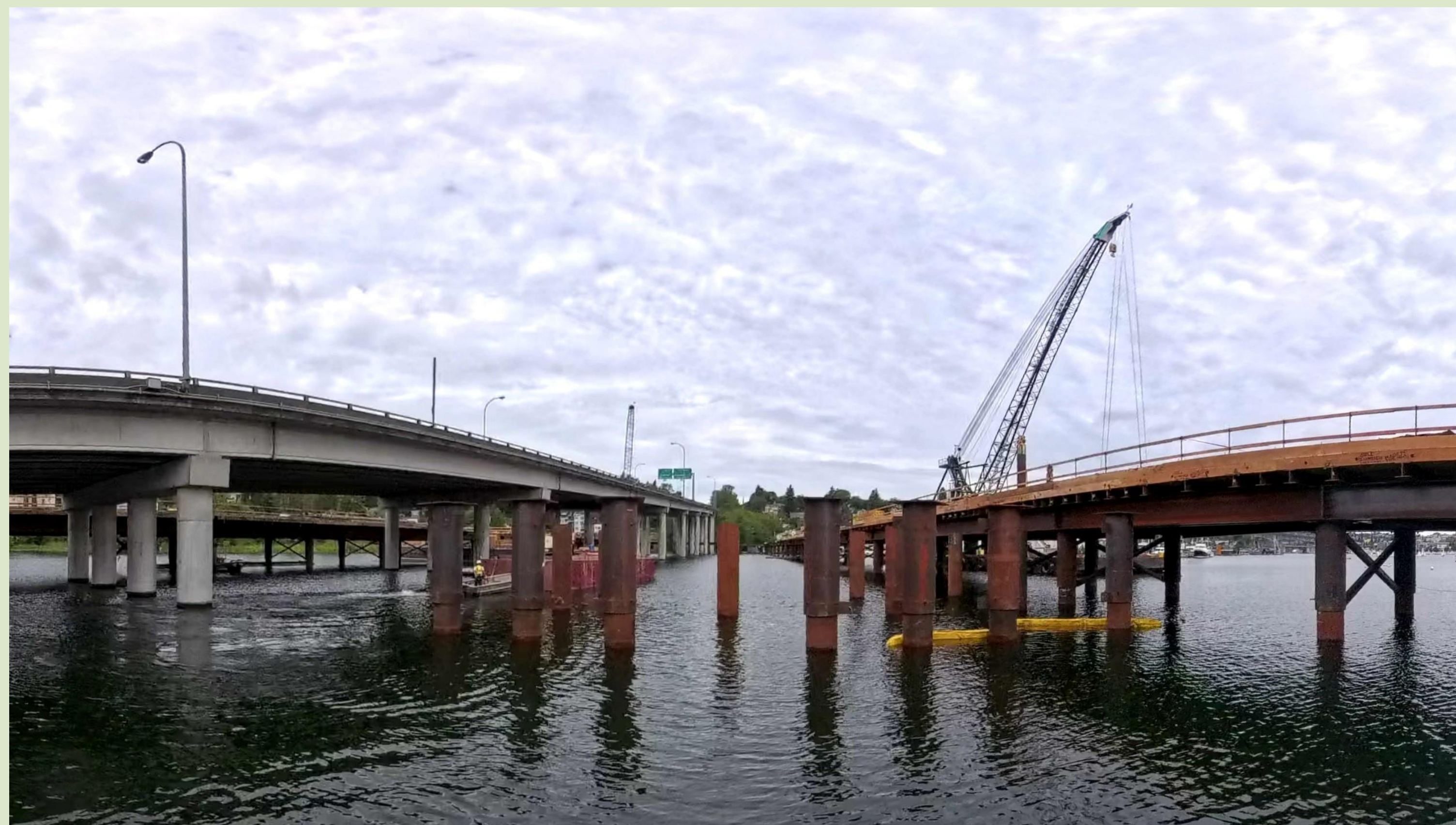
These steel piles have been driven in Portage Bay and cut to the correct height. They will support the temporary work trestle.
