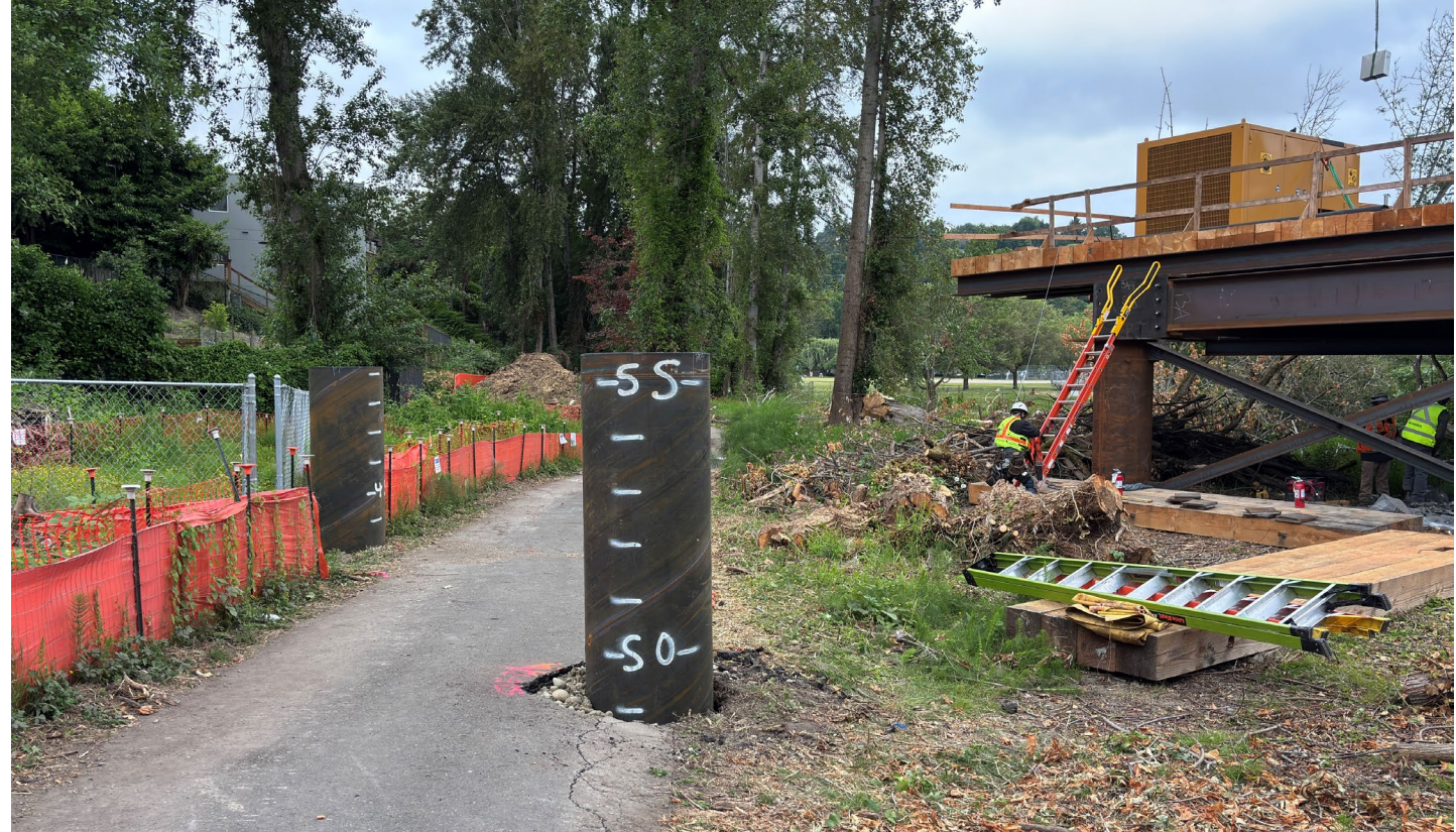
A pair of piles that will support the temporary work trestle on the Bill Dawson Trail (June 2025)
