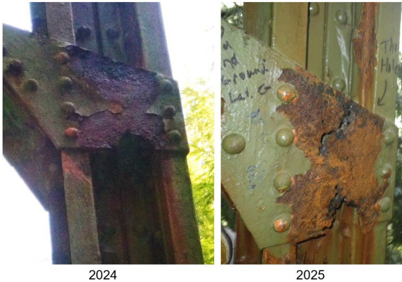
Figure 16. Bridge gusset plate
