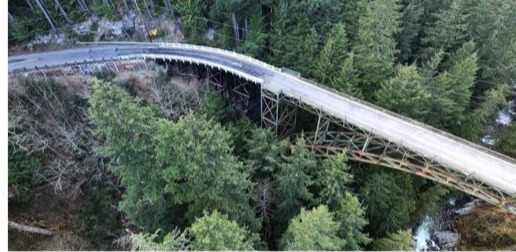
The SR 165 Carbon River Fairfax Bridge is a steel truss bridge supported by a lattice work of steel beams and columns. This recent aerial shows the rusting areas on the steel truss portions underneath the bridge deck.
