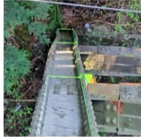
This steel support column on the bridge is bent in two directions and is starting to buckle. This compromises the column's ability to carry weight from above.
