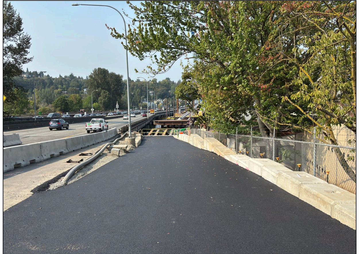
New pavement on the temporary haul road (looking west). This haul road will provide access to and from the north work trestle via Montlake Boulevard.
