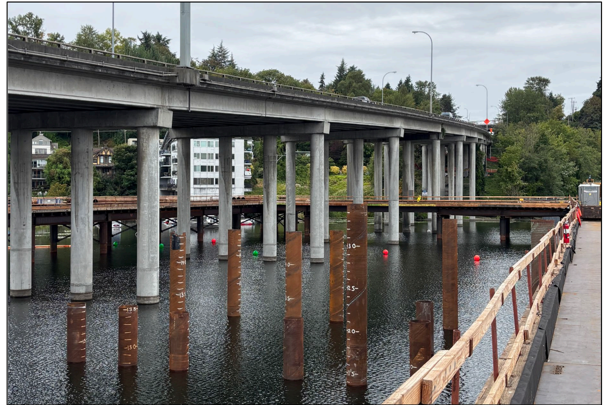
An area north of the Portage Bay Bridge where additional piles will be installed in Season 2 to extend the temporary work bridge (August 2025)
