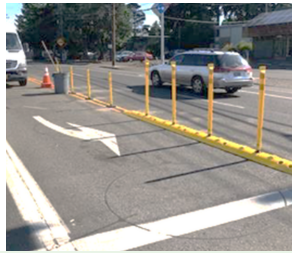
Hardened Centerline/Turn Hardening
